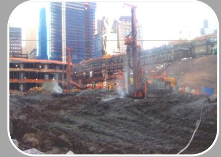
USA , Ground Zero - DTH hammer drilling (Im-Loch-Hammerbohren)
